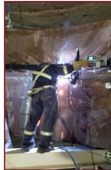
Figure 5: FCAW-G automated welding
