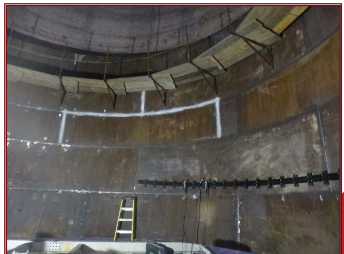
Figure 6: Ore bin with engineered scaffolding.
