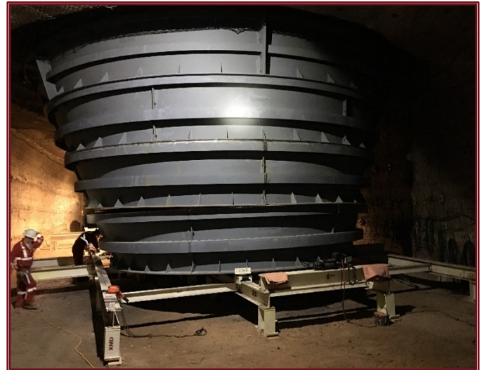
Figure 4: External fitting and alignment of ore bin
