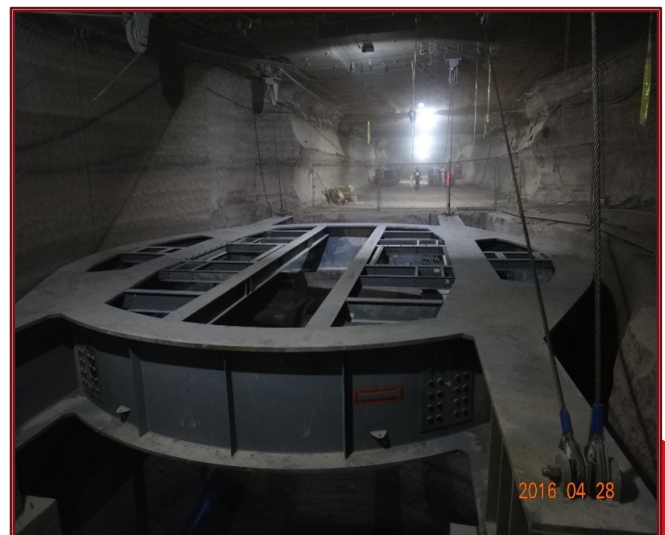
Figure 3: Completed upper hitch beam
